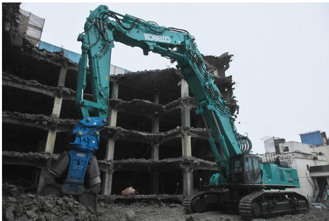
Picture 1 - Example high reach demolition machine
