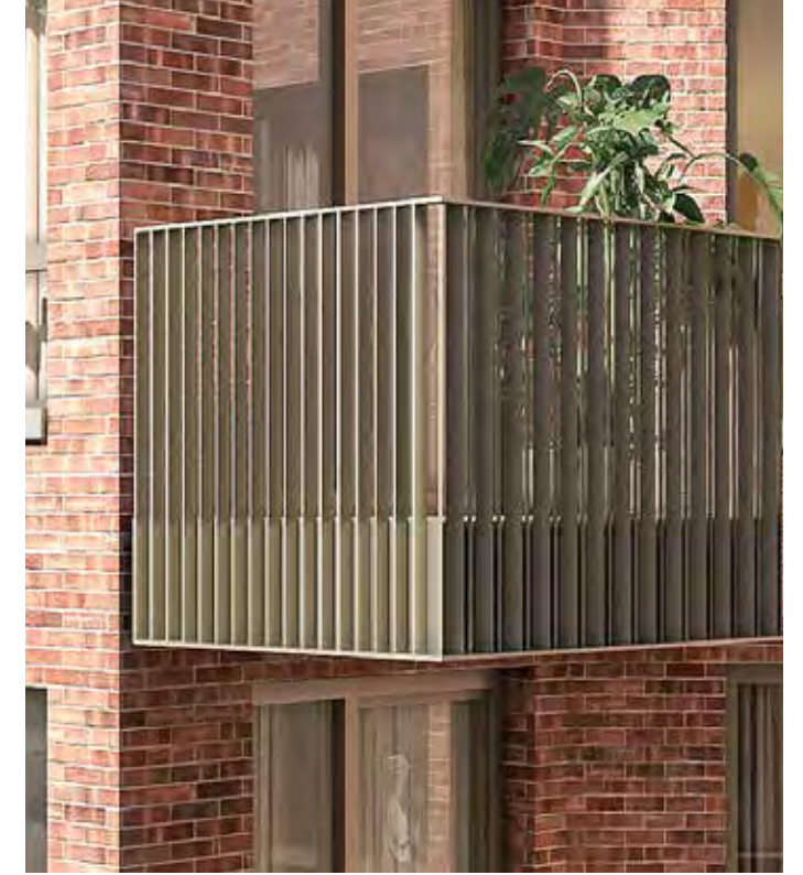
■ Painted metal guarding with angled metal flats for privacy and painted metal handrail and soffit
