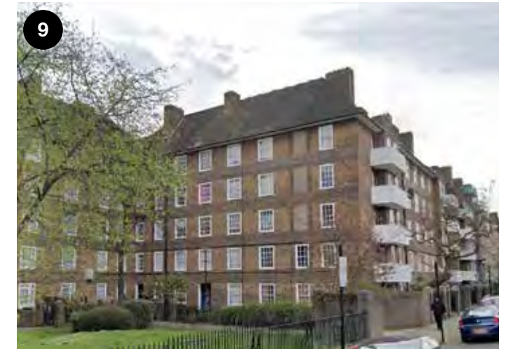
9 Biddlestone Road Estate
